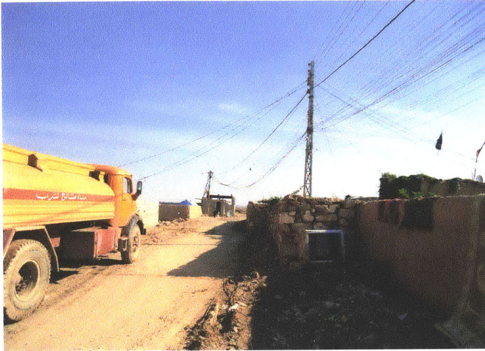
IMPROVED WATER SERVICES, ELECTRICITY, AND CONSTRUCTION
