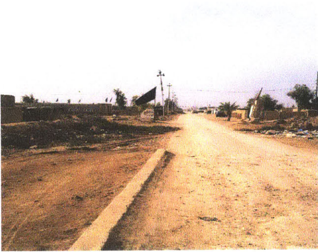
COMPACTED GRAVEL ON ROADS
