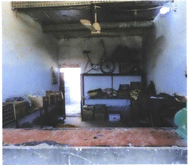
DURABLE STEEL ROOF INTERIOR
