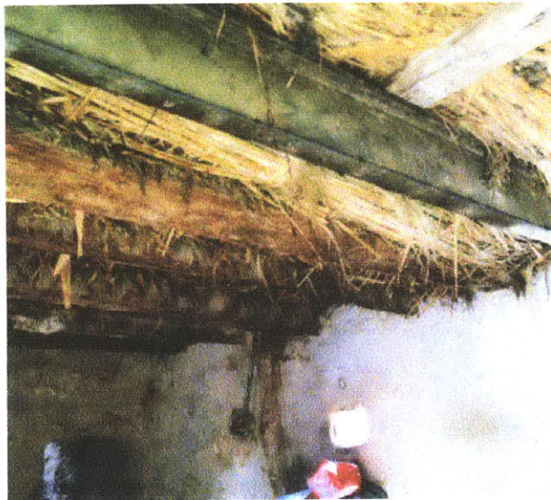
TYPICAL ROOF INTERIOR
