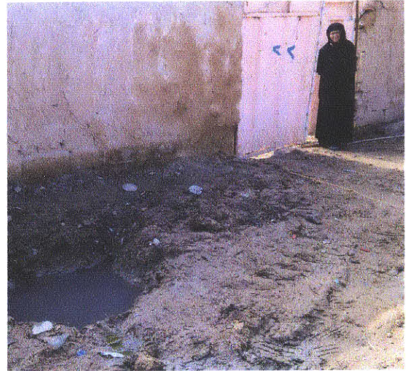
DRAINAGE OPENING FROM HOME TO ROAD
