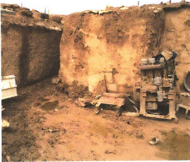
NON-DURABLE MUD STRUCTURE
