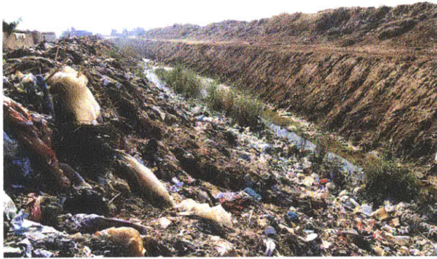
IRRIGATION CANAL FILLED WITH SOLID WASTE
