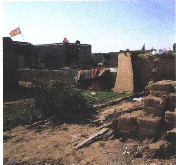
ROAD FOR STORAGE OF CONSTRUCTION MATERIALS
