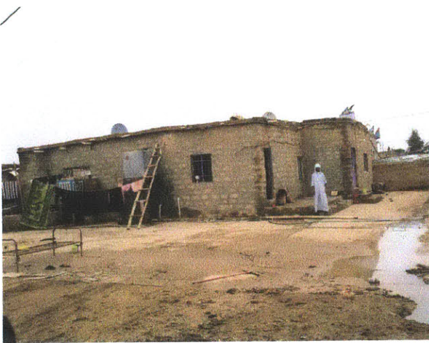
PERSONAL DRAINAGE CANAL
